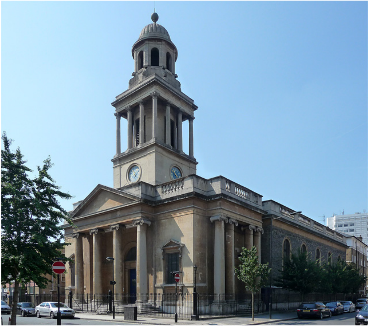
The building in Cosway Street
